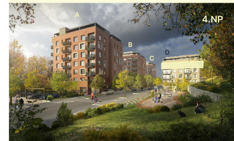
Pohled na dům / Building View
