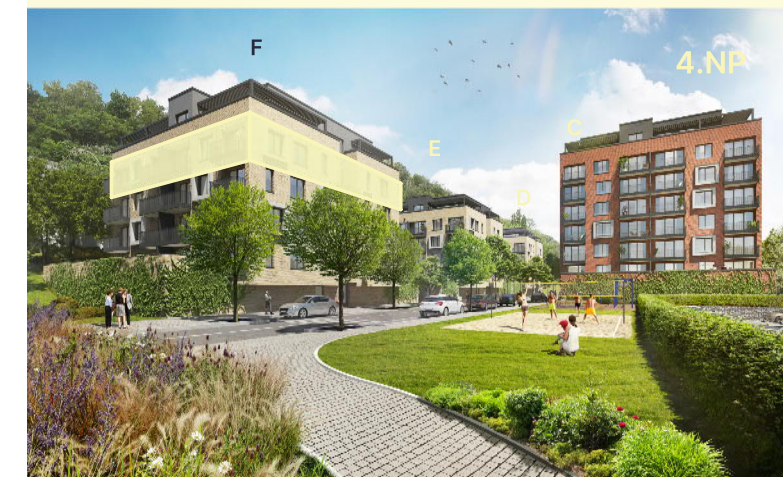
Pohled na dům / Building View
